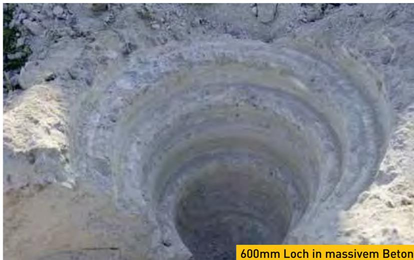
600mm Loch in massivem Beton
