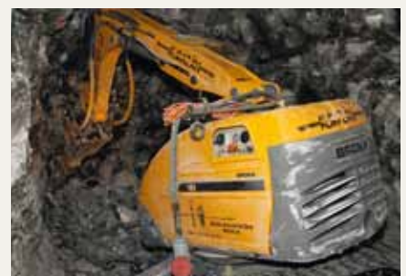
Excavating drainage tunnel. Brokk 180 with SB 202 in Spain.
