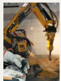
Breaking bathroom tiles. Brokk 50 with breaker SB 52 in Uppsala, Sweden.
