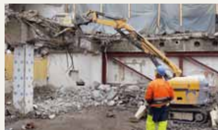
Concrete crushing with Brokk 400 and CC 700 in France.
