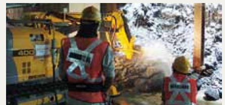
Brokk 400 with SB 552 demolishing a diaphragm wall in Singapore.
