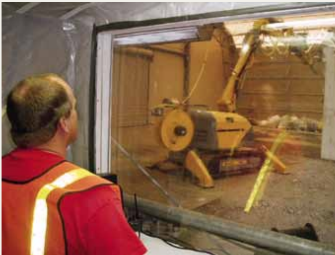
Demolishing a hot cell behind acrylic glass. Brokk 330 with SB 450 in USA.
