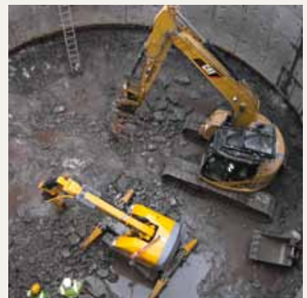
Excavating vertical shafts. Brokk 400 with SB 552 in Glasgow, UK.
