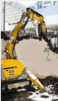
Concrete crushing with Brokk 180 and CC 420 in Hong Kong.
