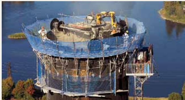
Brokk 330S demolishing a chimney in Norway.
