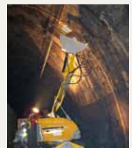
Making cuts in railway tunnel. Brokk 180 with wall saw in France.
