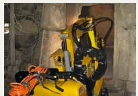
Entering a kiln inlet sec- tion with Brokk 50.
