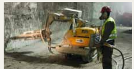
Anchor drilling. Brokk 180 with drill in Spain.
