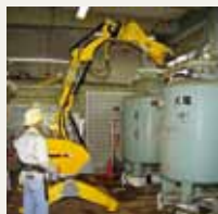
Cutting pipes. Brokk 180 with steel shears in Japan.
