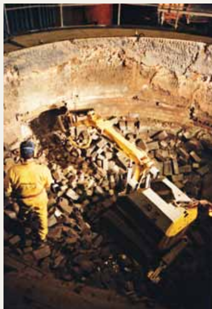
EAF removal of bricks. Brokk 150 with bucket.
