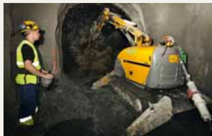
Breaking out for emergency exit. Brokk 330 with SB 450 in France.
