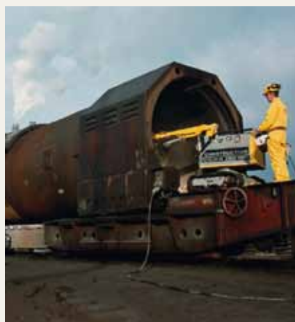
Brokk 150 entering a torpedo ladle in Linz, Austria.
