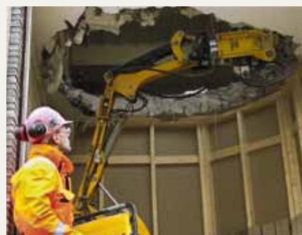
Demolishing ceiling with Brokk 90 and CC320, Norway.
