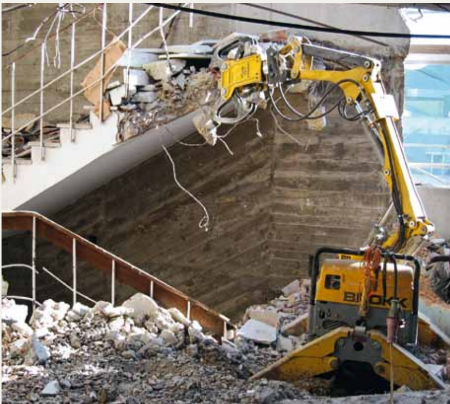
Demolishing staircases with Brokk 90 and CC 320 in Frankfurt, Germany.
