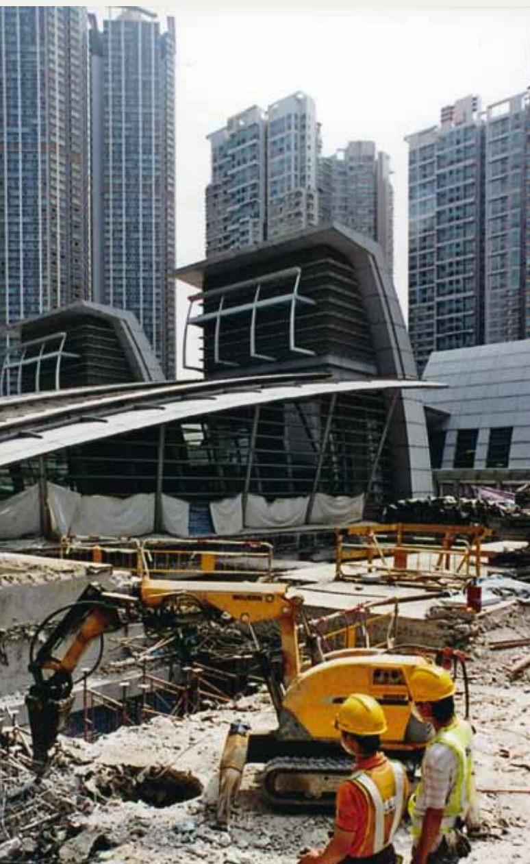
Concrete breaking with Brokk 180 in Hong Kong.
