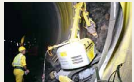
Excavating safety niches. Brokk 330 with SB 450 in Ireland.
