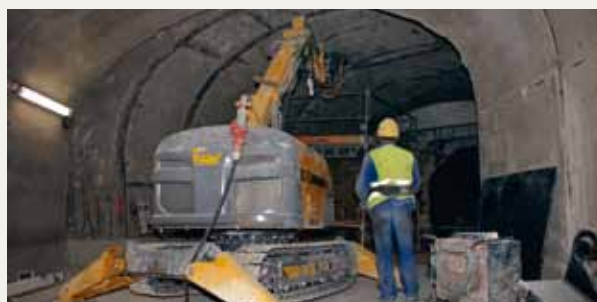
Enlarging existing tunnel and excavating new tunnels. Brokk 400 with SB 302 and side angling device in Paris metro, France.
