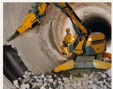
Breaking out brick lining. Brokk 330 with SB 300 in Gotland, Sweden.
