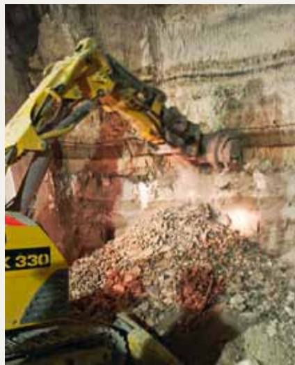
Excavating safety niches. Brokk 330 with concrete cutter in Paris, France.
