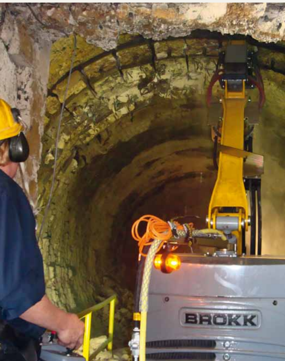
Tearing down bricks in a cement kiln. Brokk 180 with SB 202 in Malaysia.
