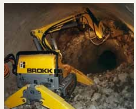
Breaking out coating. Brokk 90 with SB 152.
